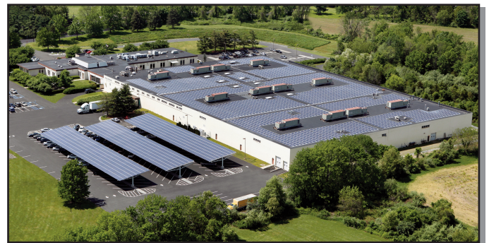
Kooltronic, Inc. Corporate Headquarters, showing approximately 4,000 solar panels in roof top array and parking lot canopies, which provide the facility with 90% of its energy requirements on any given day.
